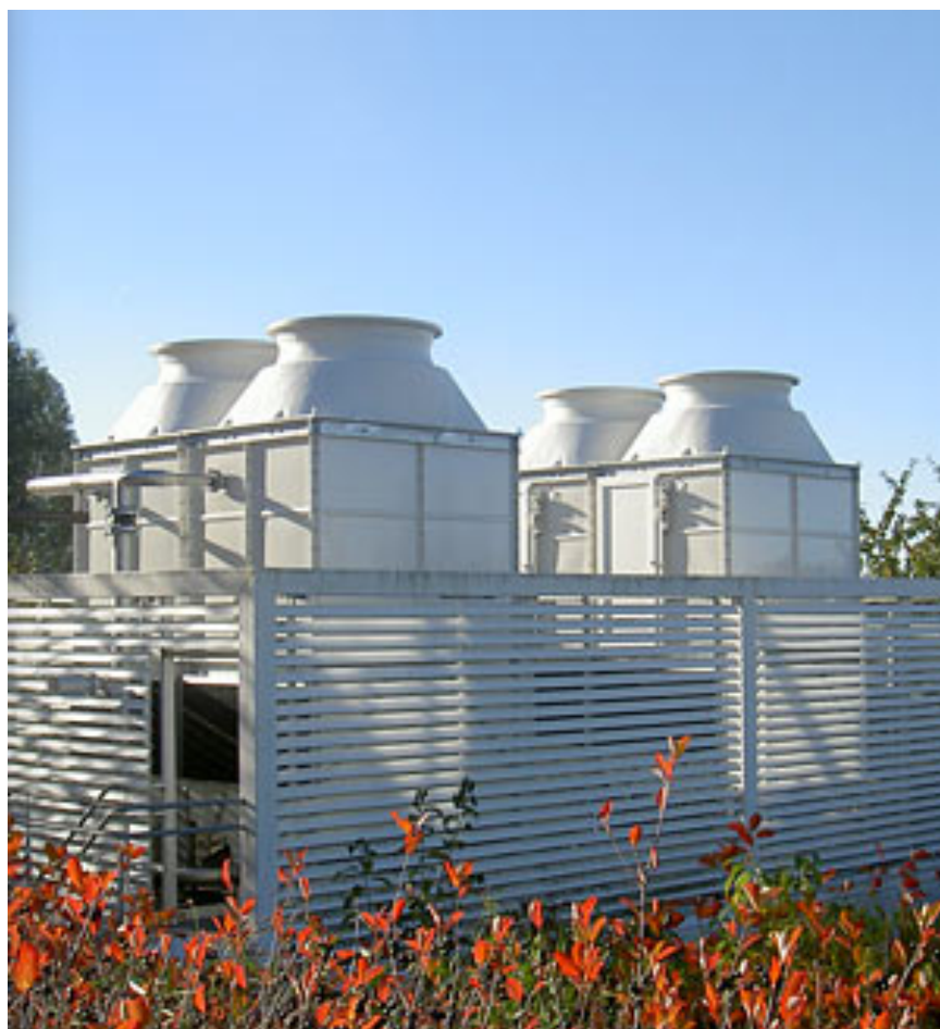
Figur 28. Modulkyltorn typ Vestas OCT05LHB02-2-120. SAS Flight Academy, Arlanda.
